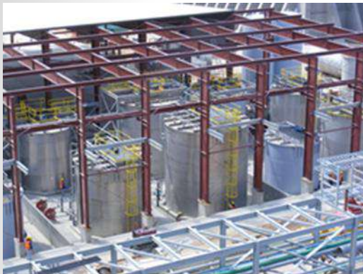
Stainless and carbon steel tanks, piping and process vessels for M3 Engineering/Gold Corp in Mexico
