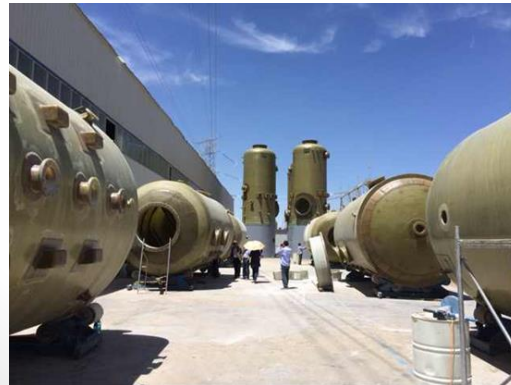
Onsite fabrication of quench towers and process vessels Hatch/QSLIC
