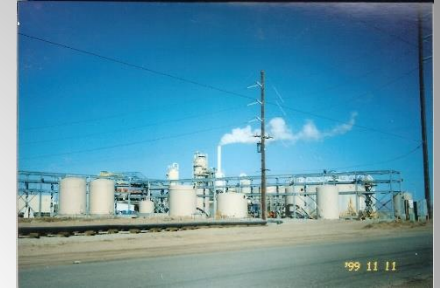
125 tanks for a zinc recovery plant
