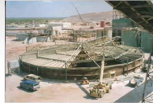
150 ft dia. hot brine thickener cover New Mexico Potash
